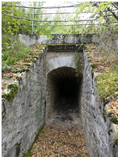
Aqueduc (PK 32k650m). Phot. Fabien Cadot IVD46_20244600085NUCA
