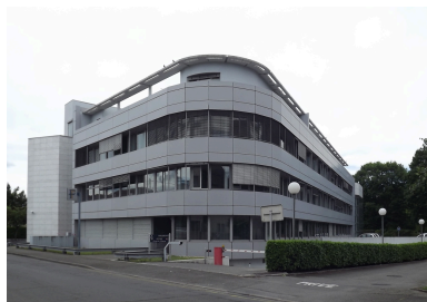
Angle sud-est. Phot. Pauline Bonnefous IVR73_20146501091NUCA
