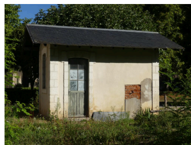
Toilettes,  levation sud-est. Phot. Guillaume Bernard, Phot. Fabien Cadot IVD46_20204602029NUCA
