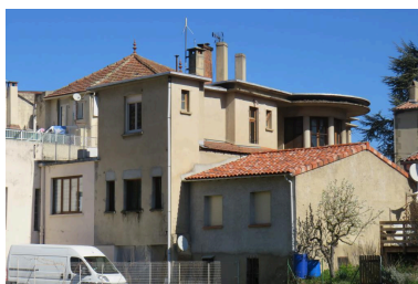
Elévation sud-ouest. Phot. Lucas Destrem IVC09160_20200900087NUCA
