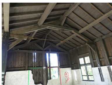
Charpente. Phot. Guillaume Bernard, Phot. Fabien Cadot IVD46_20204602098NUCA
