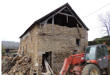
Elévation nord. Phot. Marion Fourcayran IVD65_20146500463NUCA
