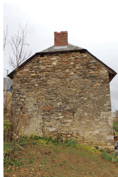
Elevation sud. Phot. Marion Fourcayran IVD65_20146500460NUCA
